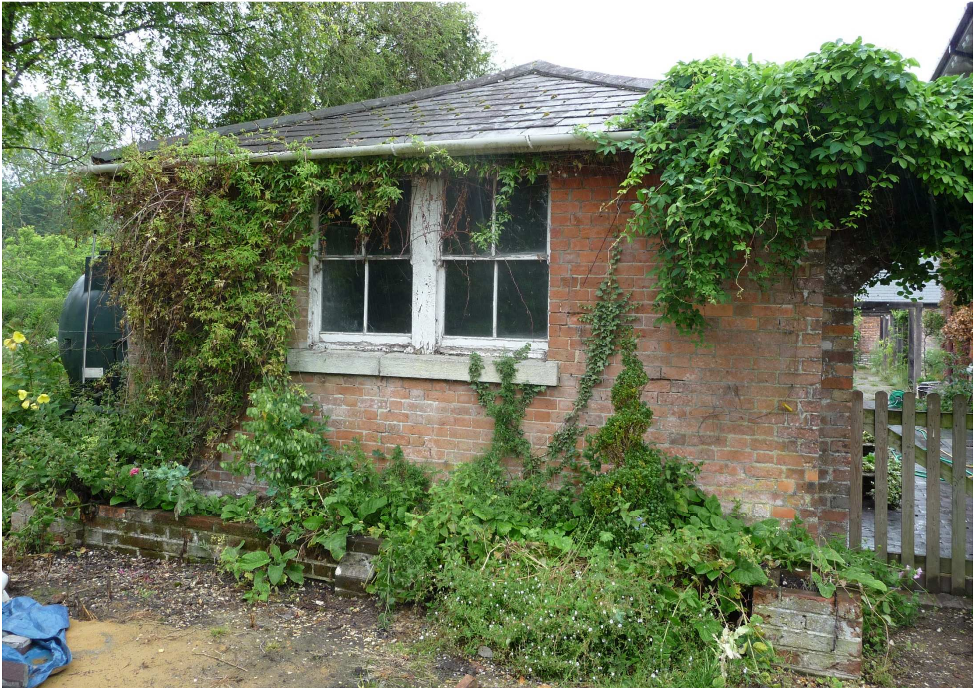
PHOTO - FRONT ELEVATION OF OUTBUILDING
